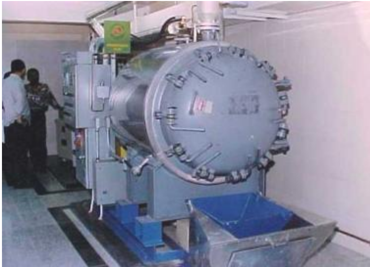
Upon installation Sept. 1999
